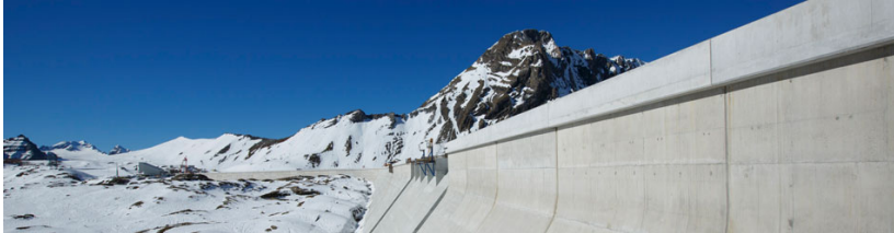
Glacial aXPo Linthal Hydroelectric Plant
